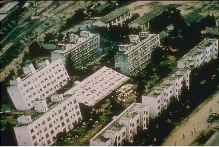
Figure 12.16 Collapsed apartment buildings in the Niigata area of Japan. The material beneath the buildings was liquefied by the 1964 earthquake. Source: DOC/NOAA/NESDIS/NCEI (1964) Public Domain view source
