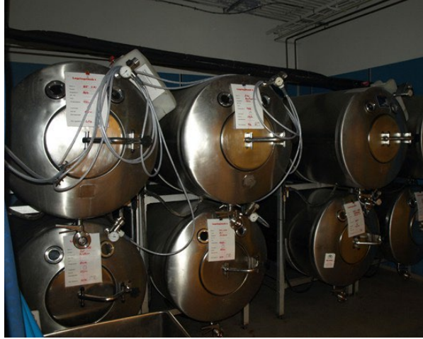
Figure 2.42 Fermentation of grape juice to make wine produces CO 2 as a byproduct. Fermentation tanks have valves so that pressure inside the tanks can be released.
