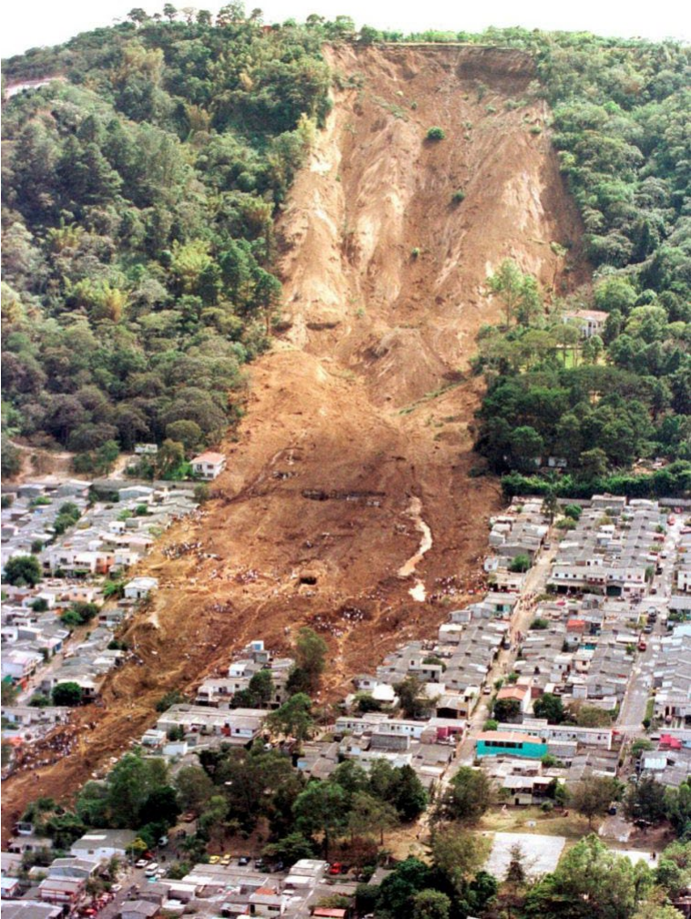
Figure 12.18 A slope gives way in a suburb of San Salvador after the January 2001 earthquake offshore of El Salvador. This is one of hundreds of slope failures resulting from the earthquake. Source: U. S. Geological Survey (2001) Public Domain view source
